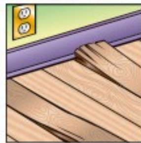
▲ loose floorboards
